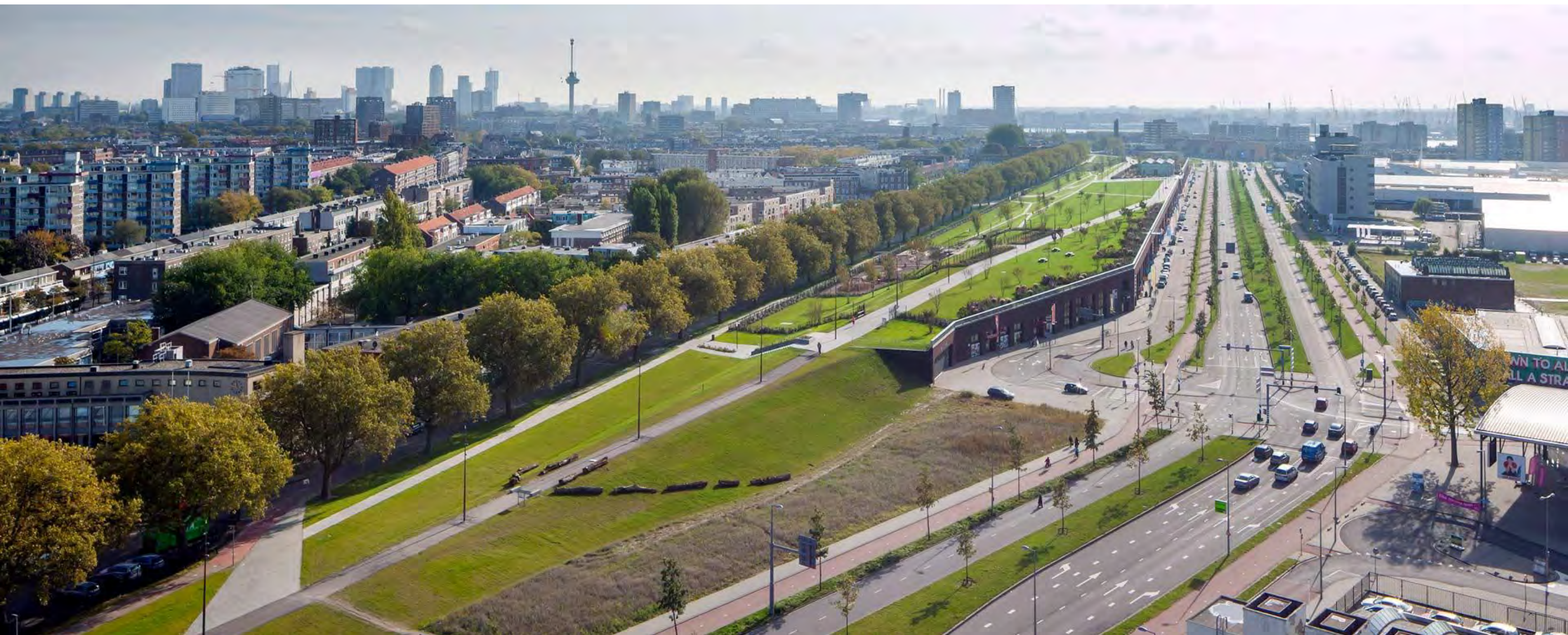
Four Harbour Roof Park. Buro Sant en Co
